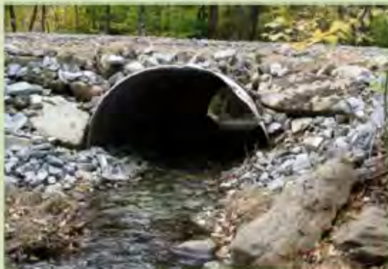
A culvert that is spanning the stream channel.
