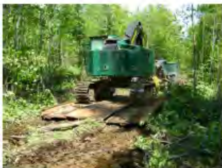
A temporary bridge.
